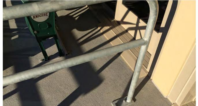
Compatibility of products at floor-to-wall transitions, detailing and drainage is vital to eliminate concerns about cure inhibition or adhesion.
